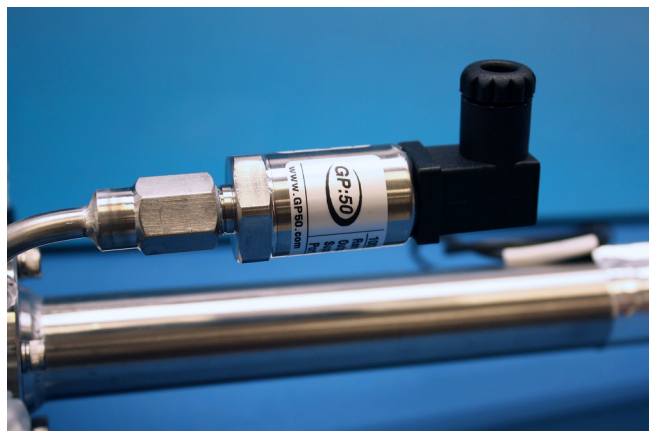
Figure B-17 Newly installed pressure sensor positioning
