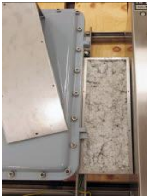
Fig 45. Unpacking enclosure insulation
